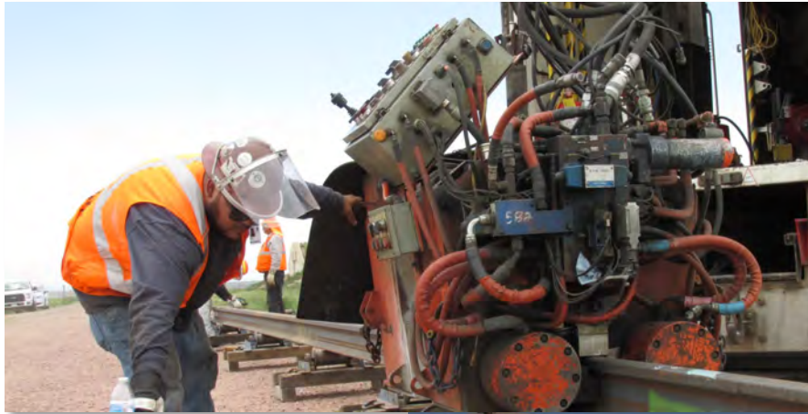
Rail welding at FAST by external contractor
