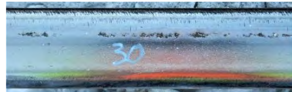
Spalling observed on high rail (above) and low rail (below)
