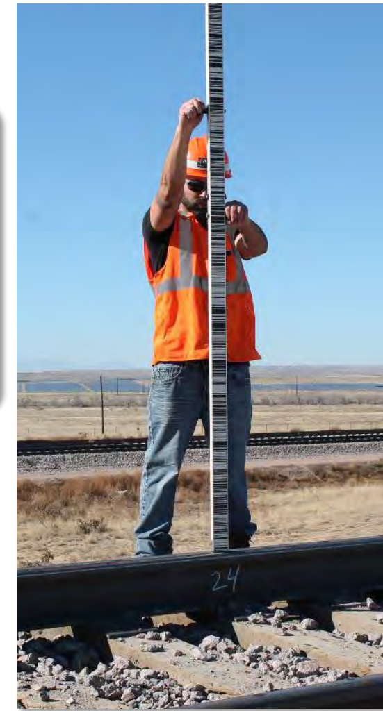
Top of Rail (TOR) survey elevations
