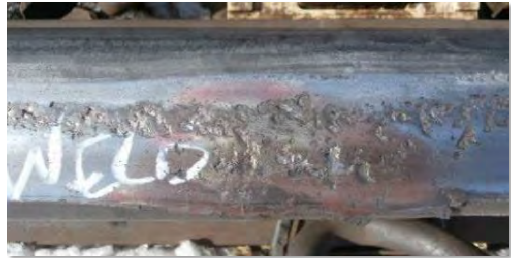
Batter of weld on low rail prior to removal
